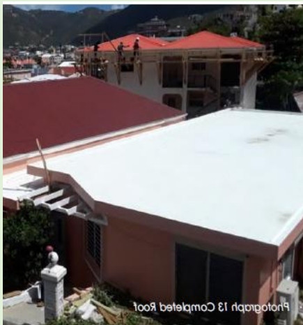
A: Roof painted white
